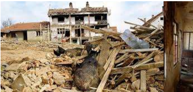
Fig.6: Damaged facilities in Kosovo (Prekaz) during the Kosovo war
