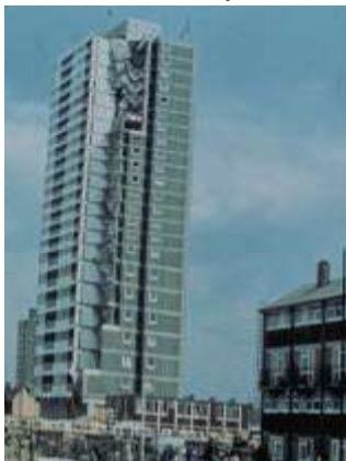
Fig.7: Progressive Collapse Ronan Point, UK, 1968[3]
