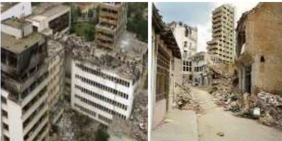
Fig. 5: Destruction of buildings with poor material compared with those of reinforced concrete
